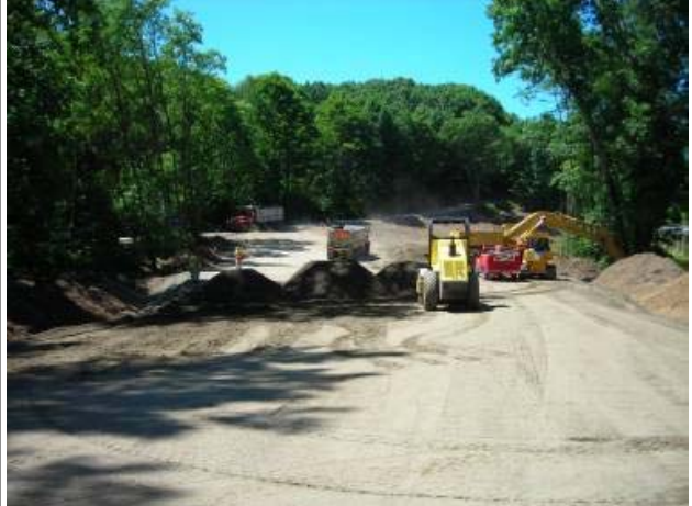
Earthwork activities to support the new pipe installation
