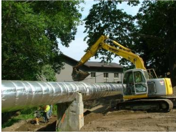
Fill materials being installed at the new downstream manhole location
