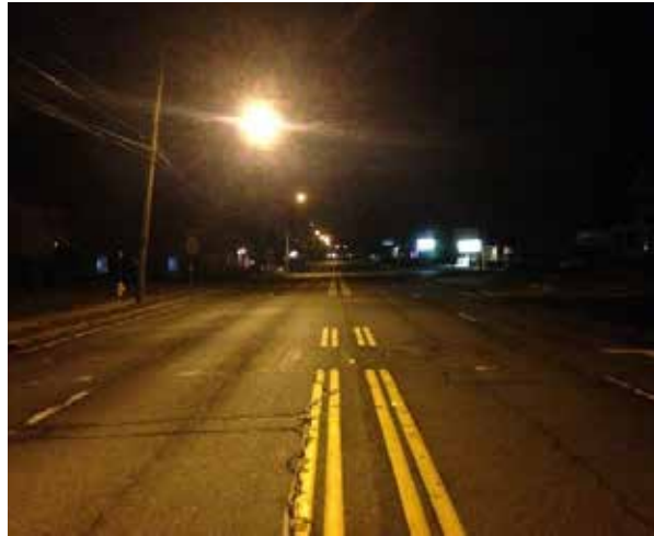
Photo looking east near Herrick Ave shows lighting on the north side of Delaware Avenue
