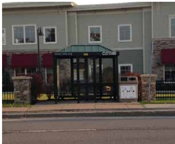
Existing eastbound station in front of Community Care Medical building (250 to 256 Delaware Ave) - One of the better equipped bus stops in the corridor.
